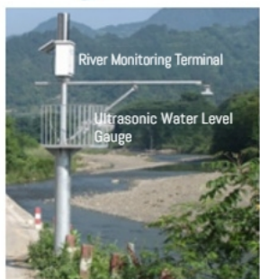
Water Level Monitoring Point (Ultrasonic)
